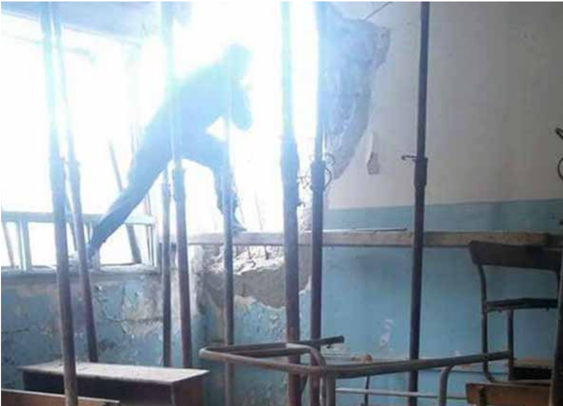
A local school being repaired in Moadamiya three months after surrender
