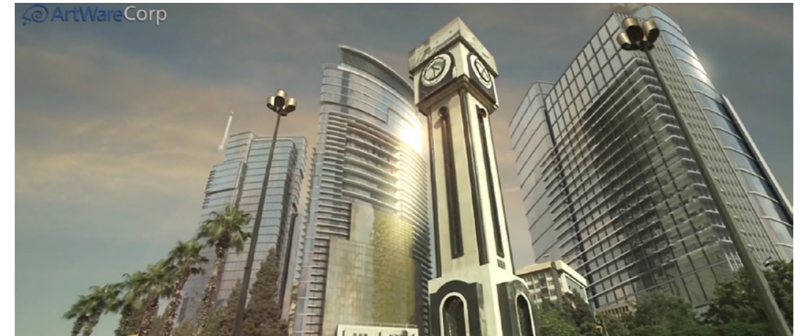
Modern buildings tower over the famous Clock Square in a reimagined Homs.
