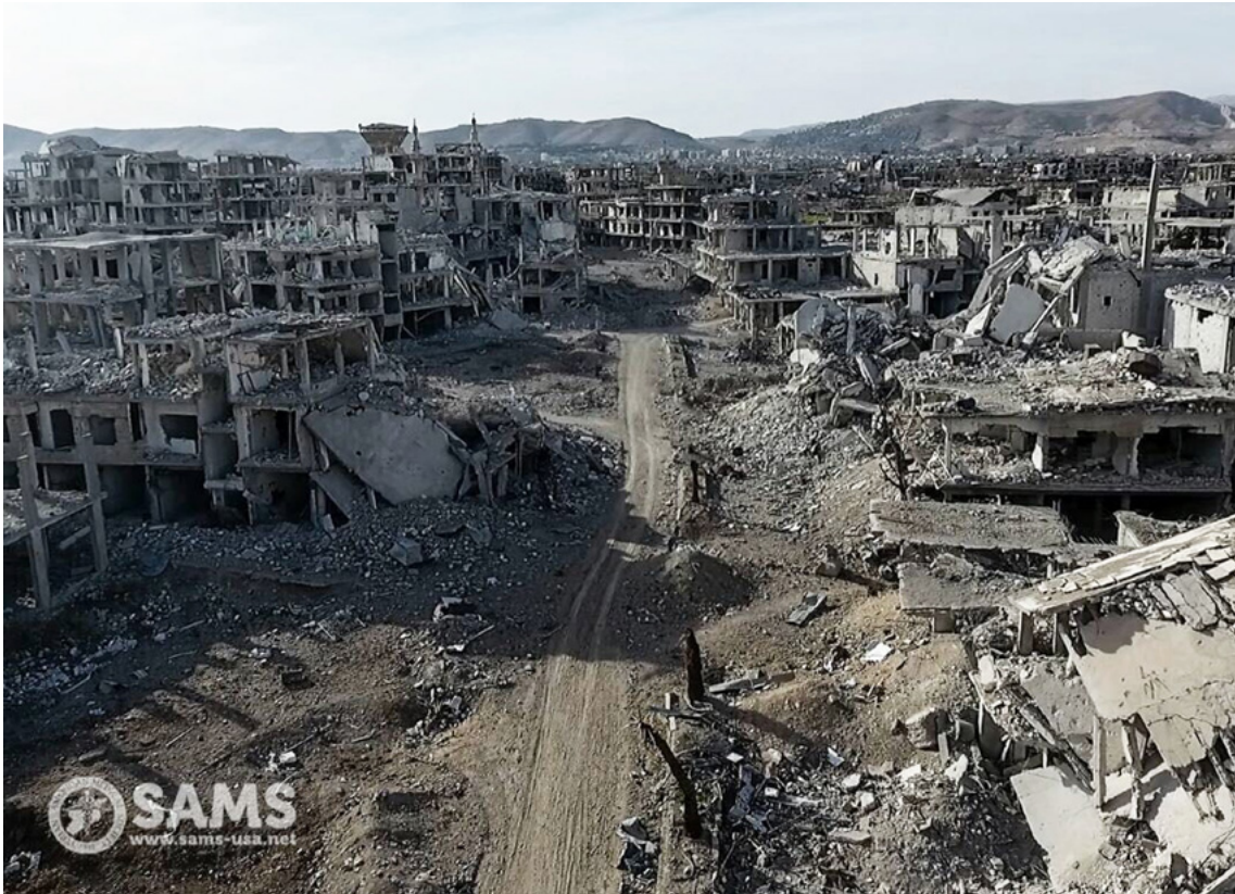
Catastrophic destruction in Arbin, 4 March 2018. Source: SAMS
