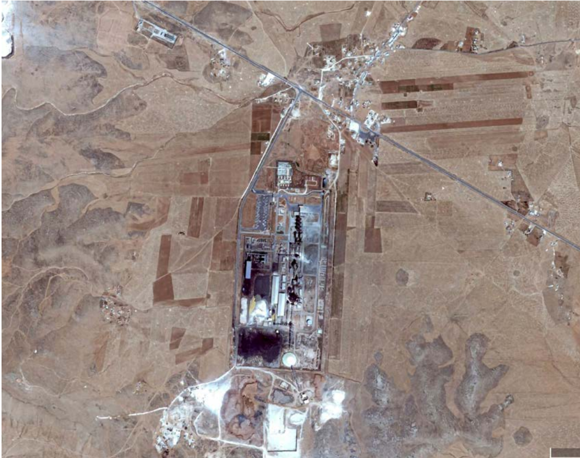
MAXAR via Google earth V 7.3.6.9345. (July 2014). Lafarge Syria Cement Factory. 36°32'34.91"N, 38°35'33.24". ( https://earth.google.com ).
