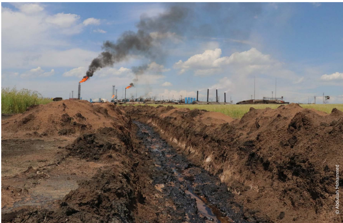
Oil waste is flowing from the Suwaydiyah refinery, April 26, 2020
