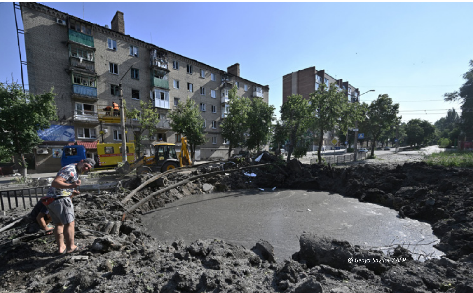
Crater filled with water after a missile struck a water pipeline in the town of Bakhmut, on July 1, 2022
