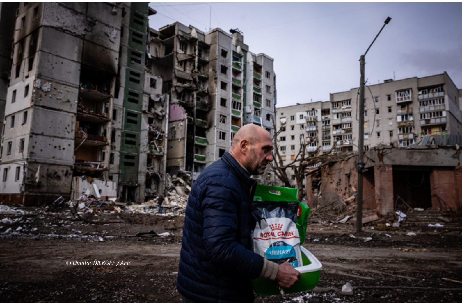
A man walks in front of a residential building damaged in shelling in the city of Chernihiv on March 4, 2022
